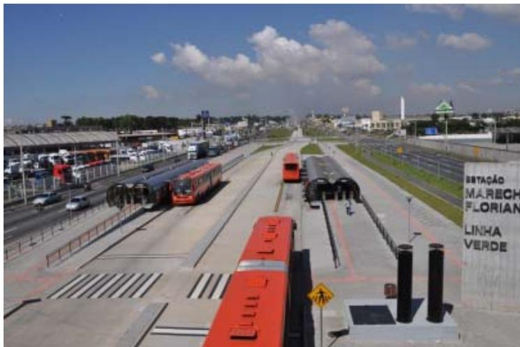
**Figure 8 Overtaking Lane at Green Line in Curitiba**
