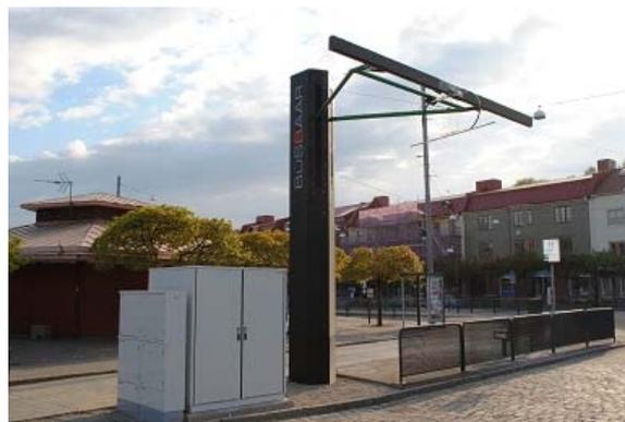
**Figure 1**The ultra fast charging station at Bus Stop in Gothenburg
