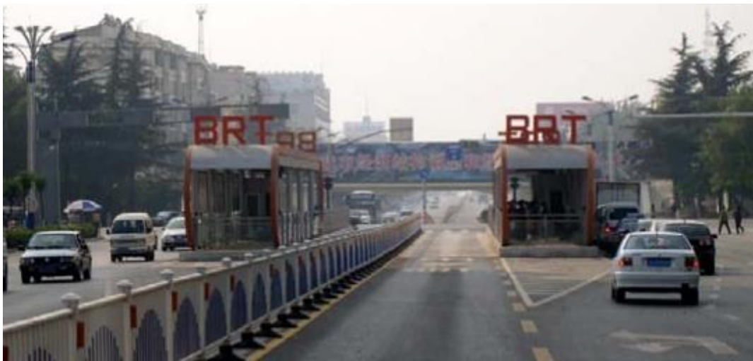
Figure 11. Zaozhuang City BRT System (source: web)
